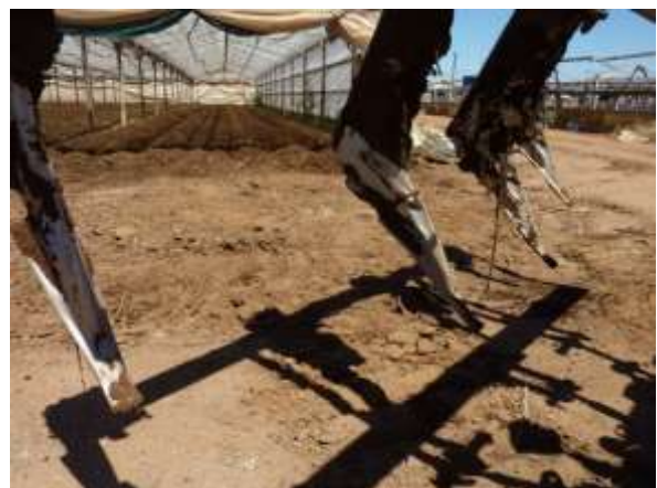
Ripping helps to improve drainage and leaching
