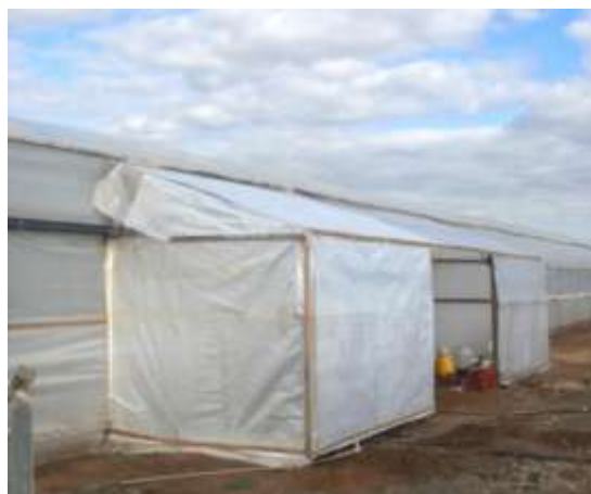
Double entry door under construction
